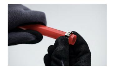
Step 2: Slip PEX pinch clamp over pipe and insert fitting.
