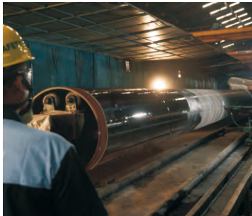
External Epoxy Coating
